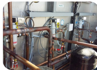
3-way valves for in-line condenser
