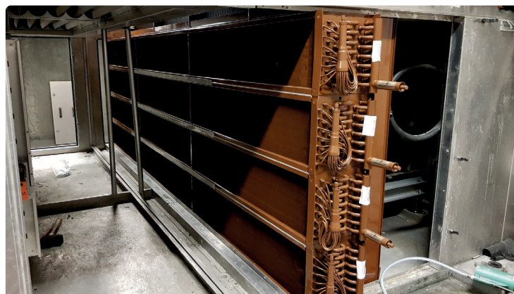
Coil with Heresite anti-corrosion protection
