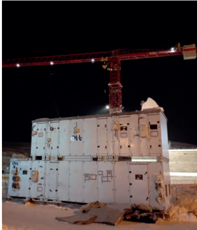
Double flow AHU
