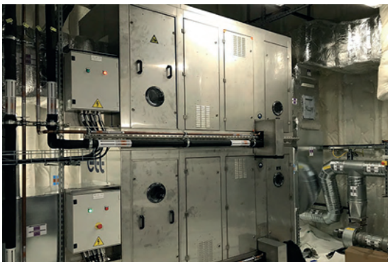
Air handling unit for pressurisation
